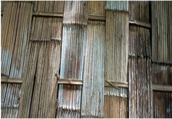
wall of the vernacular house
